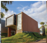
THE VICTORY BY ANDAMAN ASSET SOLUTION
