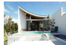
THE TRINITY VILLAGE PHASE 2 BY ANDAMAN ASSET SOLUTION
