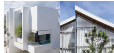
THE RESIDENCE BY ANDAMAN ASSET SOLUTION
