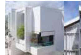
THE RESIDENCE BY ANDAMAN ASSET SOLUTION
